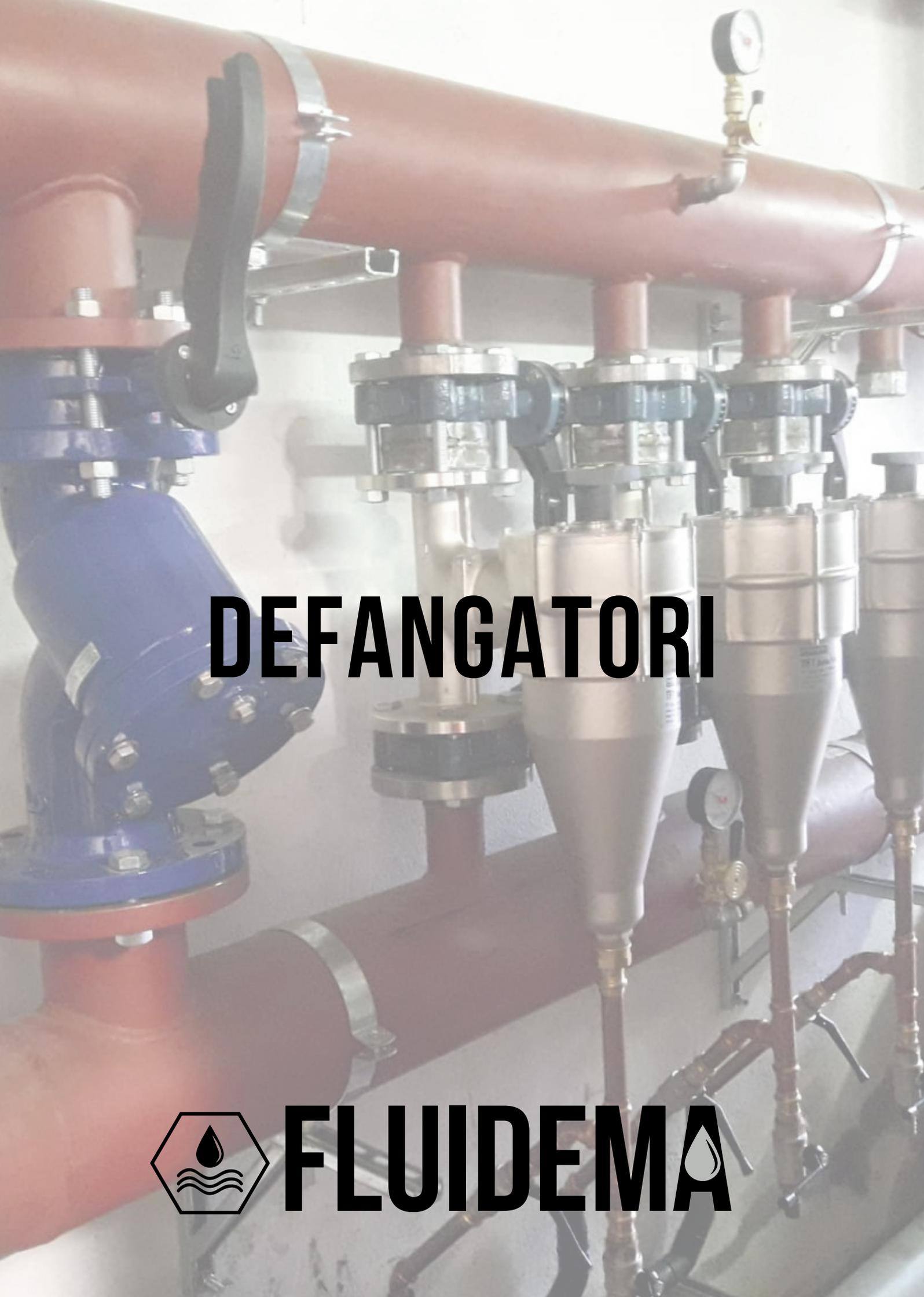
A photograph of an industrial piping system. A large horizontal pipe runs across the top. Below it, several vertical pipes lead to conical defangators. A blue valve is visible on the left. The background is a plain wall.
